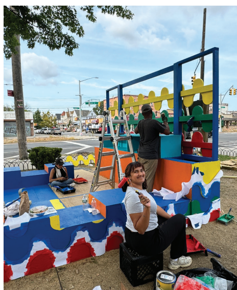
Painting the structure
